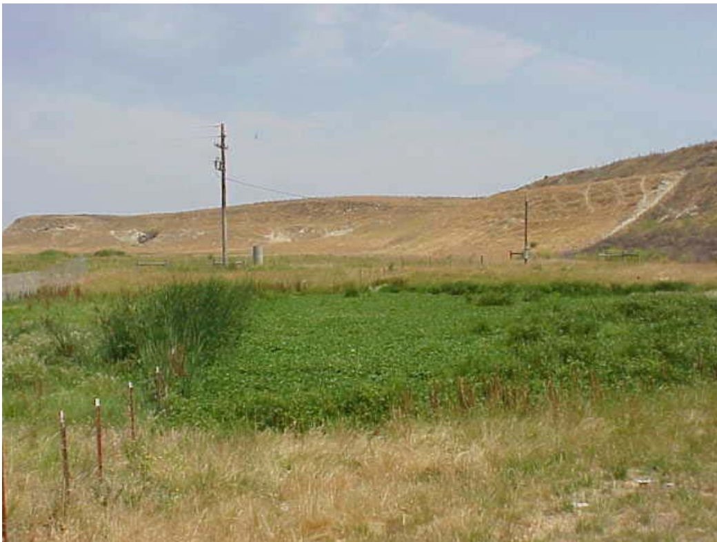
Photo 6: DK outfall maintenance basin.
