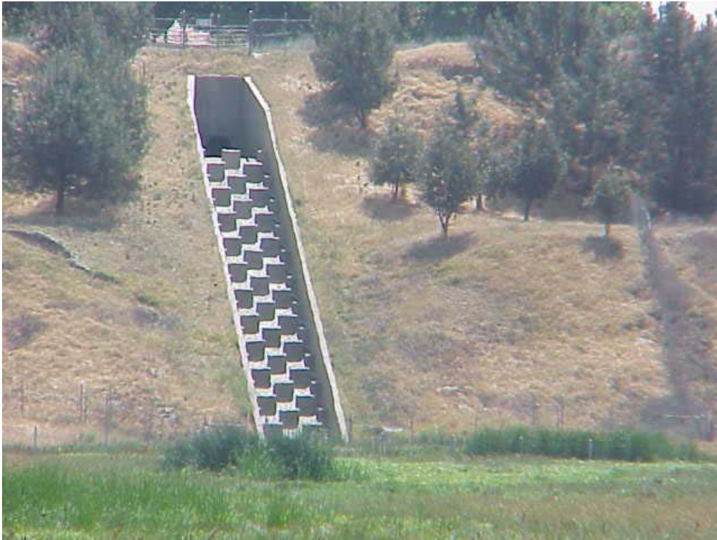
Photo 5: Fresno Metropolitan Flood Control District's DK outfall into maintenance basin.
